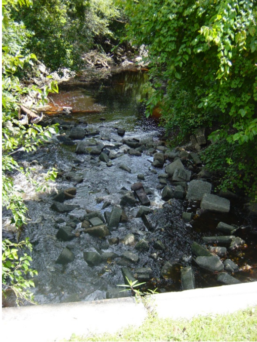
Pictures show the need for bank restoration. Fill in has been done with pieces of concrete but erosion is present in many locations.
